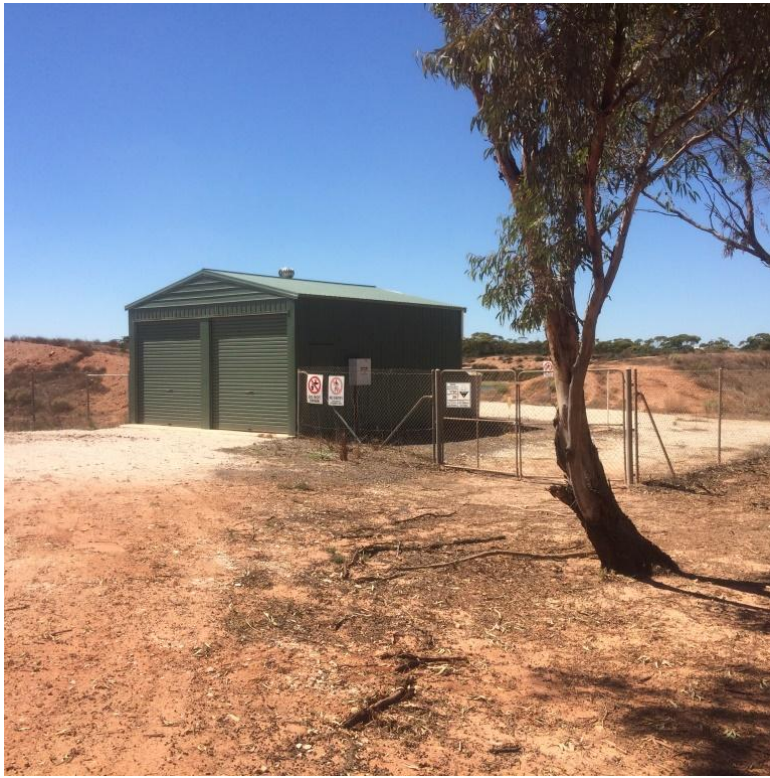
Re-use Pump Shed, Filter and Disinfection Unit: at installation time
