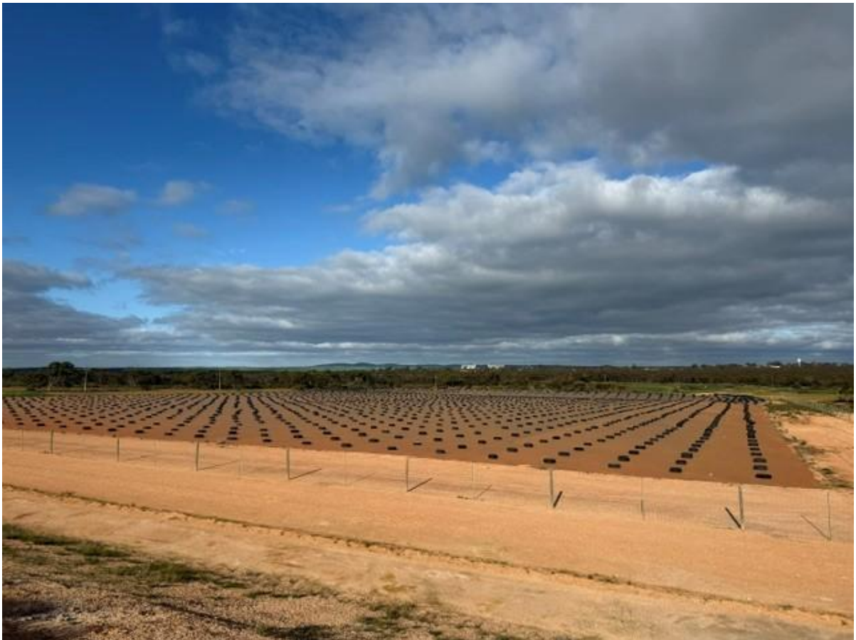
4 Ha Stormwater Harvesting Liner complementing Roora Dams
