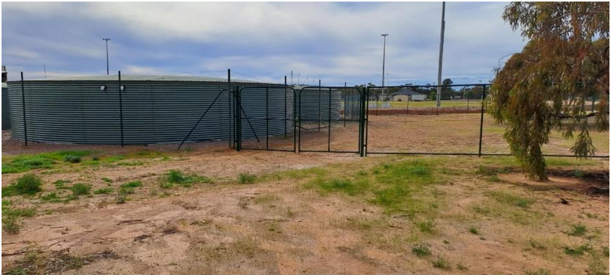
CWMS Treated Wastewater Storage Tanks at Town Ovals
