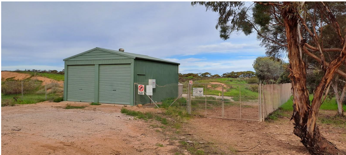
Pump Shed 16 years later: excellent condition (well-maintained)
