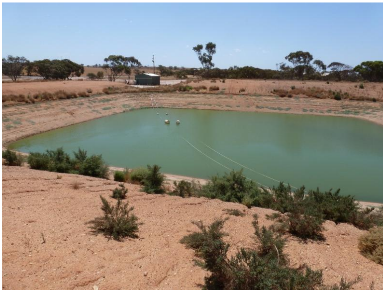
Winter Storage Pond between Facultative Lagoon and Re-use Pump Shed
