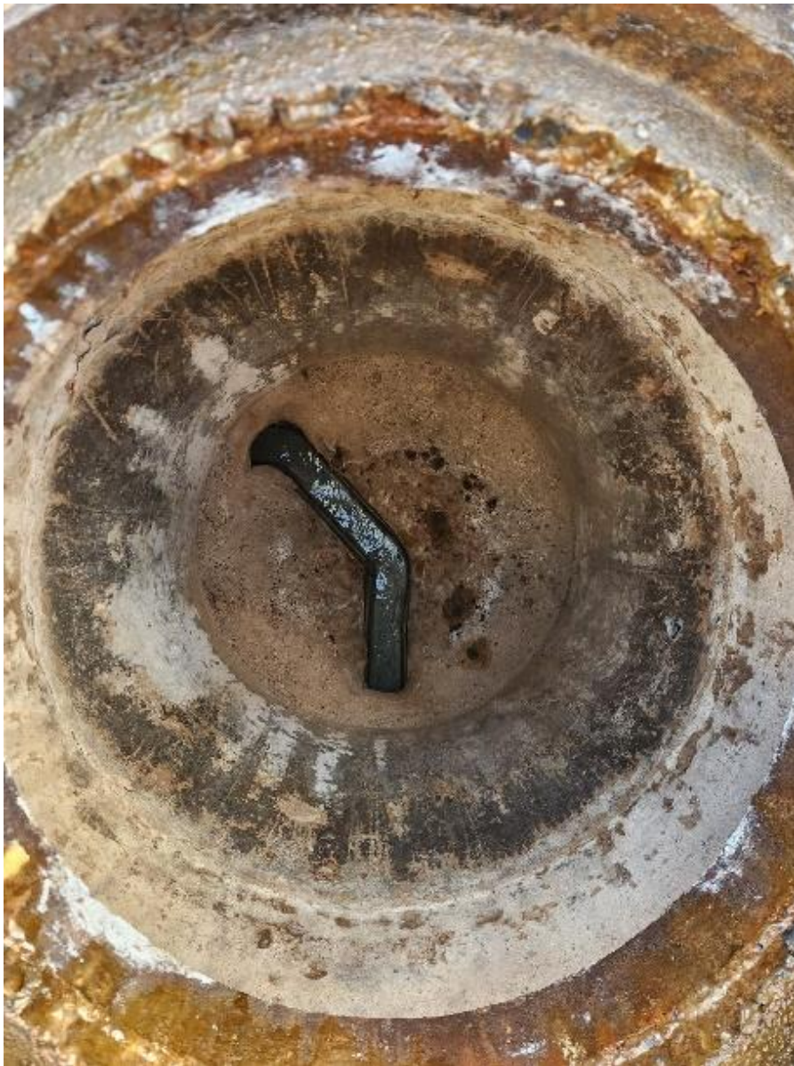
Manhole sump prior to remediation
